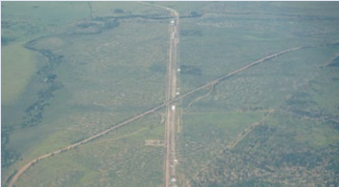
The 200km rail line to the Carmichael mine under construction
